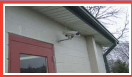
Exterior Camera Installation
